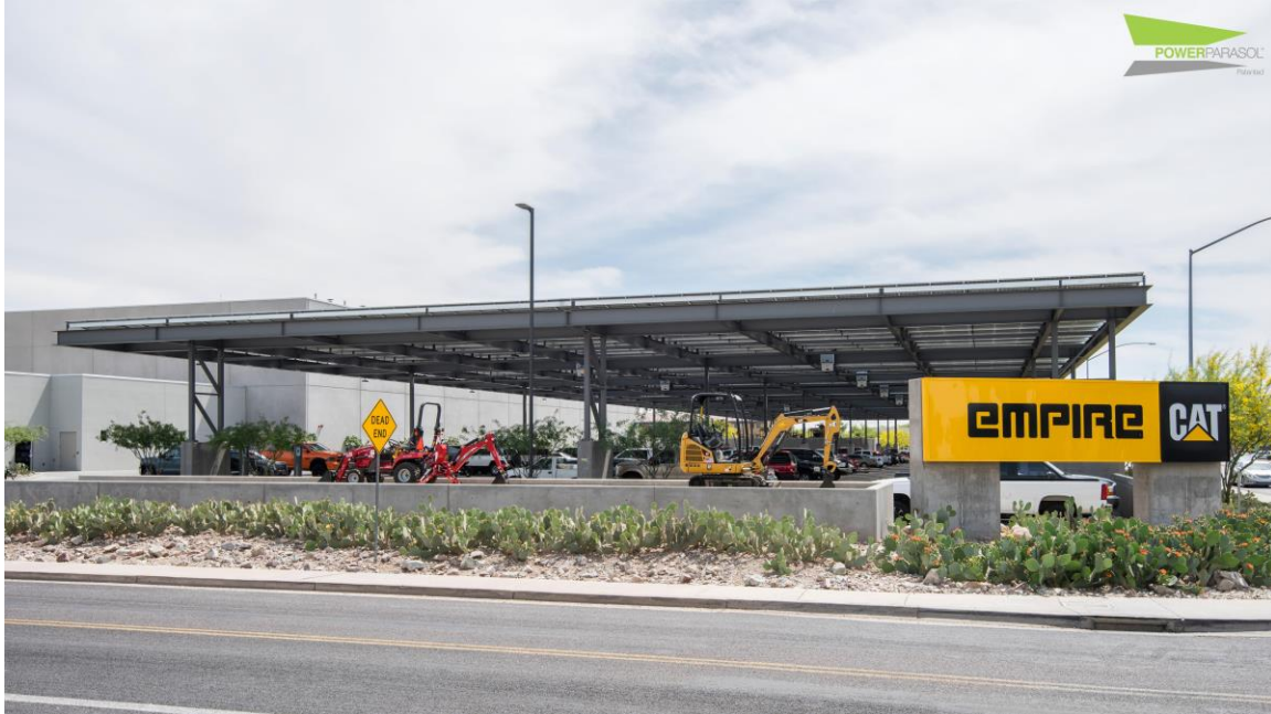
PowerParasol at the Empire Renewables Headquarters in Mesa, AZ.
